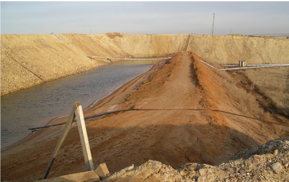
Collector pond for the pregnant gold solution between the operating heap and dam.
